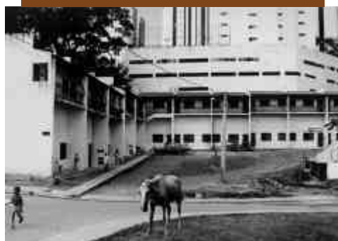
Community after the urbanization improvements
